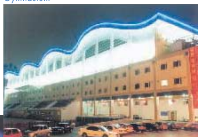
Blue light-beam illumination in the Haidian Gymnasium
