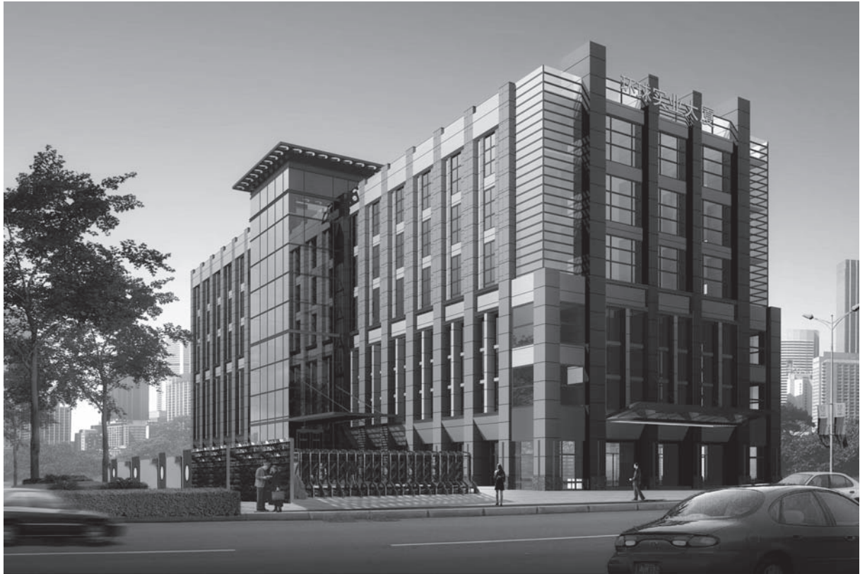
Picture of headquarters building
