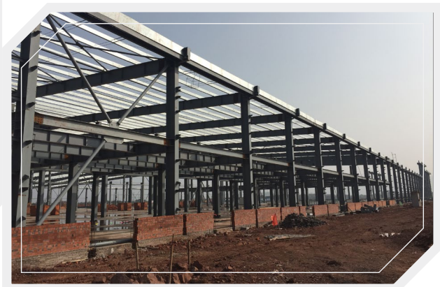
The plant of Zhejiang Forever New Energy Limited is under construction
