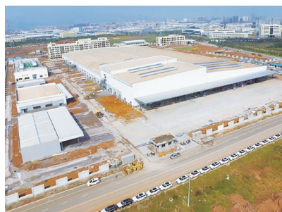
All of the major construction works have been completed
