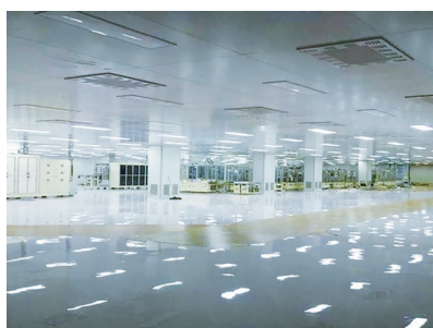
Interior of Main Building
