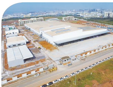
All of the major construction works have been completed
