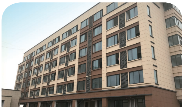
The new administrative building of Zhejiang Forever New Energy
