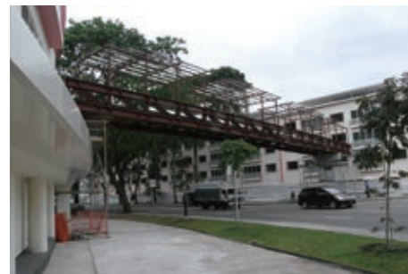
Constructing the Link Bridge
