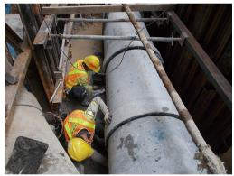
Installation of concrete pipes for sewerage system
