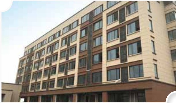
› The administrative building of Zhejiang Forever New Energy
