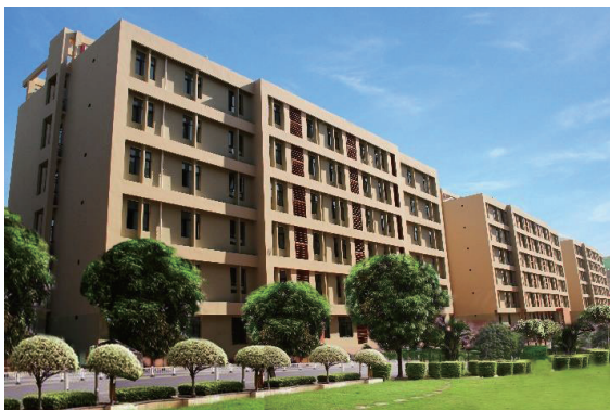
Environmental enhancement on campus site
