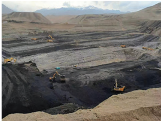
Excavation and separation works by the construction team
