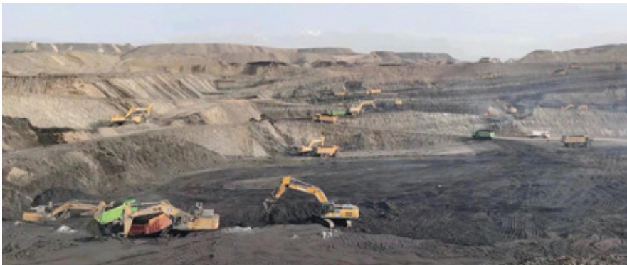
The construction team excavates and removes the soil
