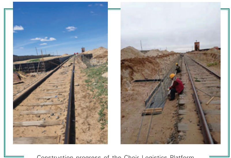
Construction progress of the Choir Logistics Platform
