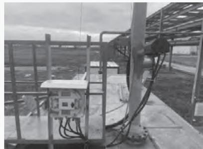
Figure: Online Monitoring System for Oil Vapour Recovery
