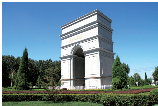
▲ Environment of campus site
