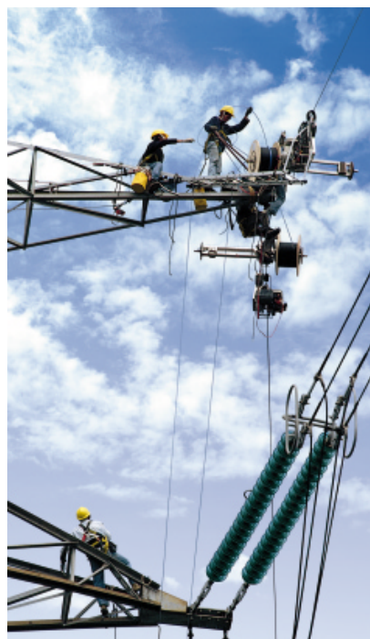
Installation work on CLP TeleCom's ChinaLink
