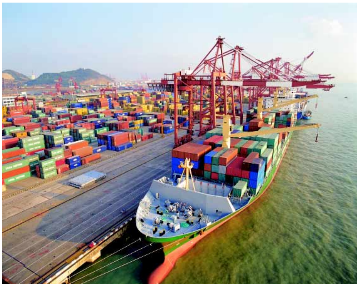
New berth at Shenzhen Kaifeng Terminal
