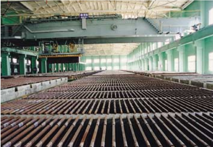
A corner of copper cathode workshop with an annual production of 200,000 tonnes
