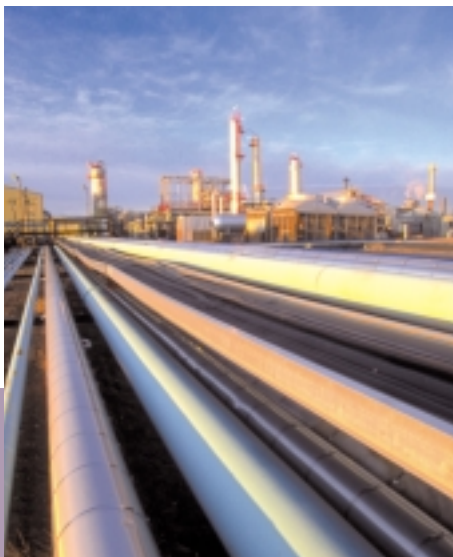
Husky's 1,900 kilometre pipeline system transports oil production from Alberta and Saskatchewan to the company's upgrading and refining operations in Lloydminster.
