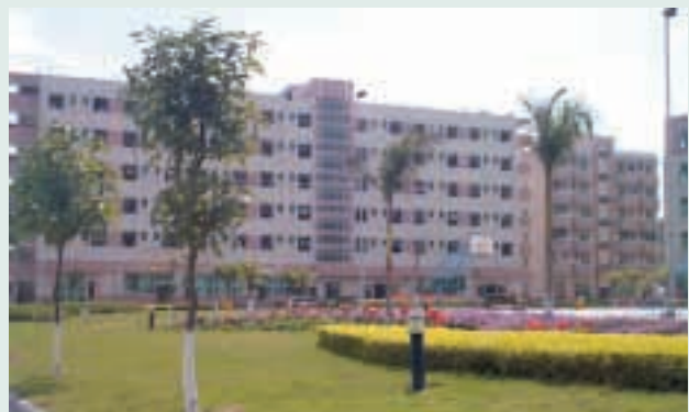
Staff Dormitory, Zhen Han Industrial City
