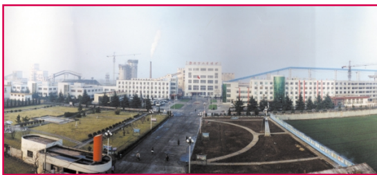
Jining II coal mine
