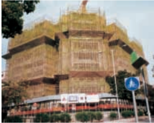
Public project – Fanling Primary Health Care Centre
