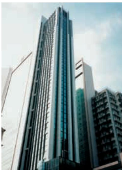
Private project-No. 40-42 Yun Ping Road, Causeway Bay
