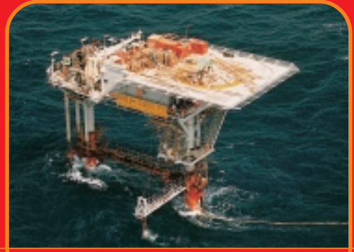
Wellhead platform C in Weizhou 11-4 Oil Field
