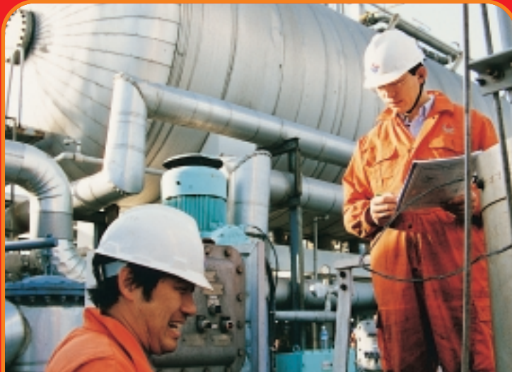
Technicians at Suizhong 30-1 Oil Field conducting oil transmission tests
