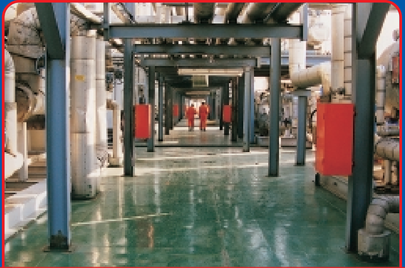
A glimpse of the Xijiang Oil Field production facilities
