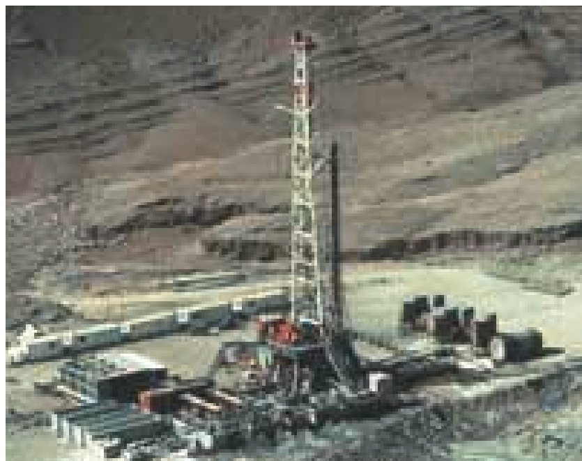
Land based drilling rig powered by Caterpillar model 3512 generating set.
