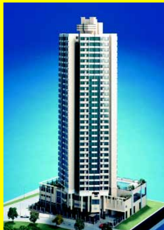
Parkview Court The commercial and residential development at Yuk Hong Street, Tuen Mun.
