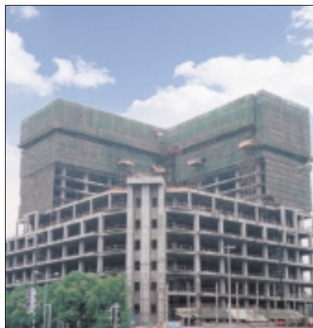
Chengdu Chuang's Centre, Chengdu, Sichuan (construction in progress)
