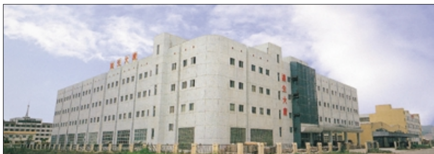
Yuen Sang Building, Danshui, Huiyang, Huizhou, Guangdong
