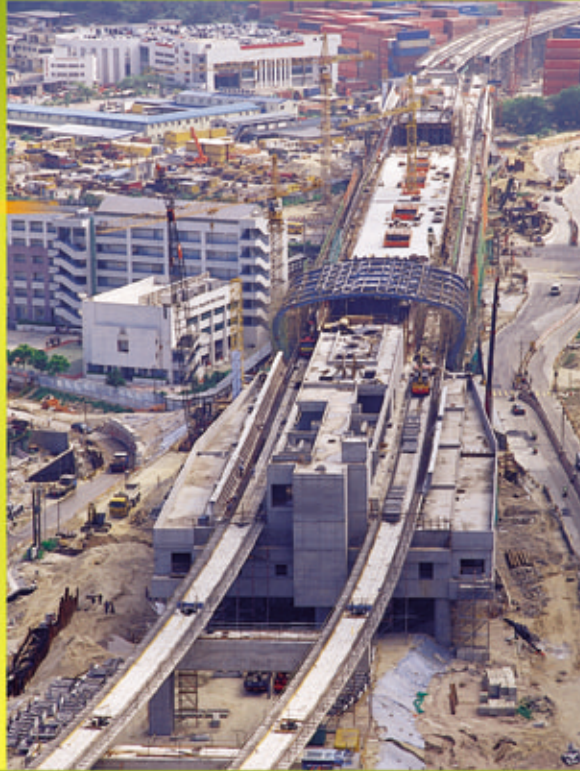
West Rail Phase 1 – Construction of Tin Shui Wai Station
