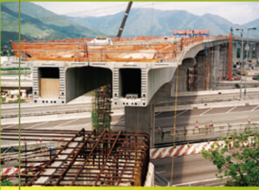
West Rail Phase 1 – Construction of viaduct from Kam Tin to Tin Shui Wai
