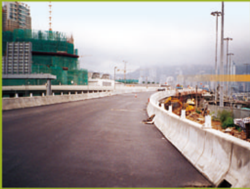
West Kowloon Reclamation Remaining Roadworks Stage 2
