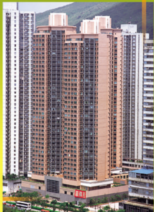
Residential Development at TWIL 17, Tsuen Wan
