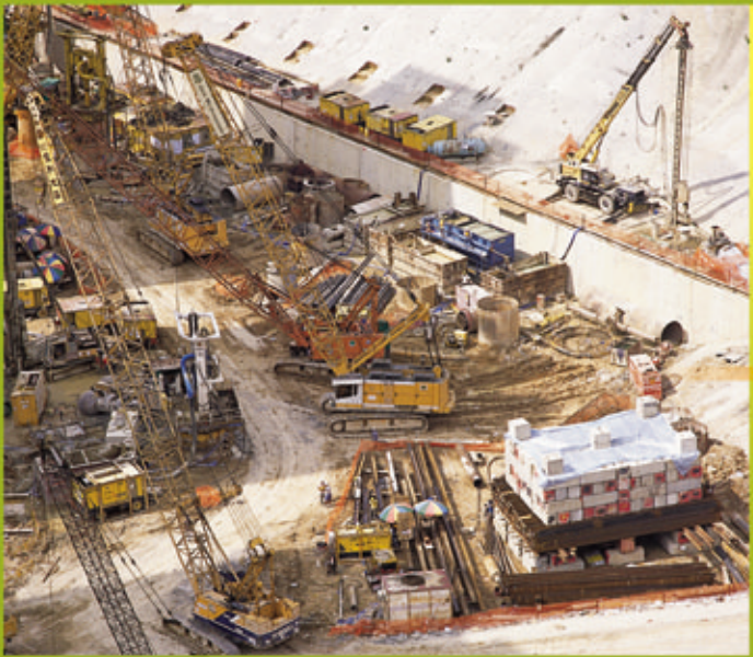
Foundation for Redevelopment of Shek Pai Wan Estate Phase 1
