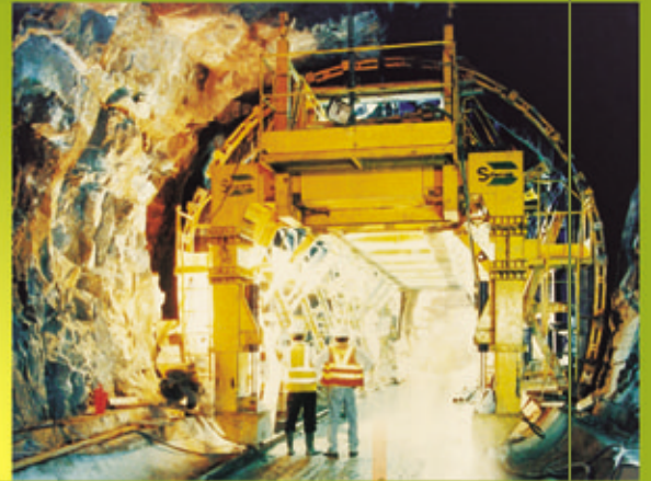
Tseung Kwan O Extension - Black Hill Tunnels
