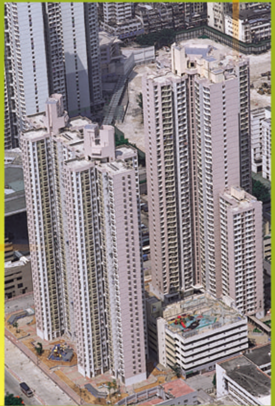
Public Rental Housing and HOS Development at Fortune Street – Phase 1, Shamshuipo
