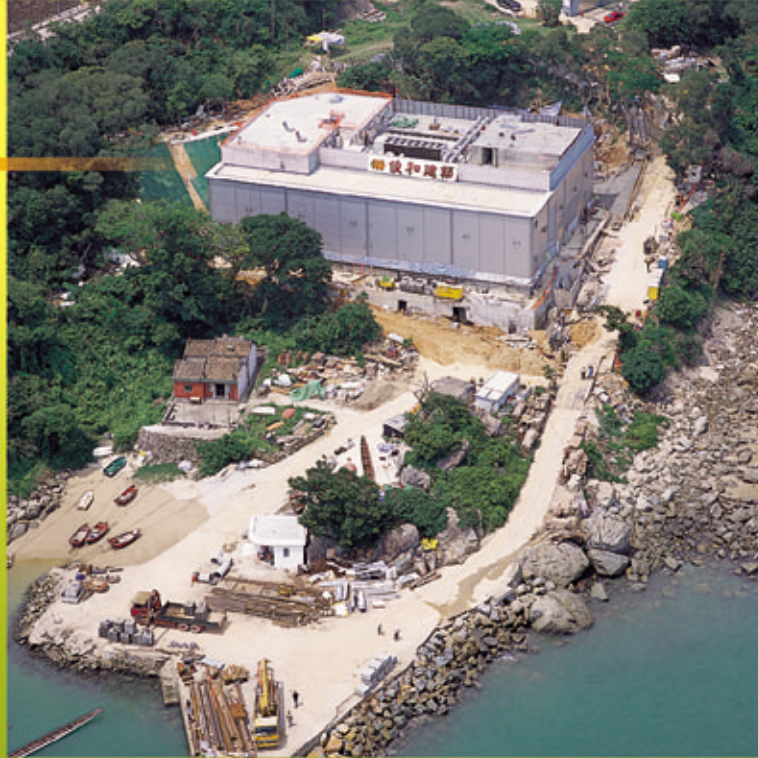
Cable Landing Station at Tong Fuk
