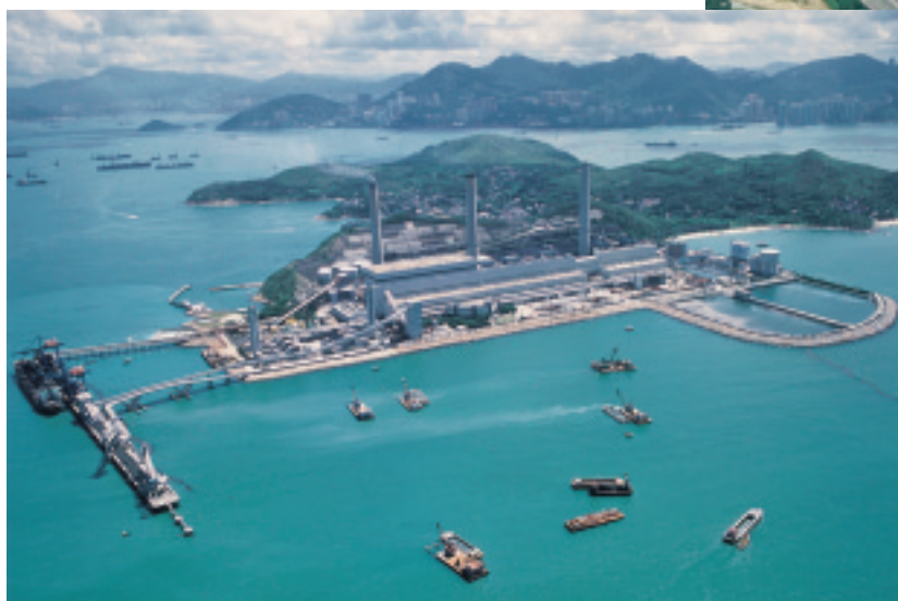
Lamma Power Station Extension Projects, Hong Kong
