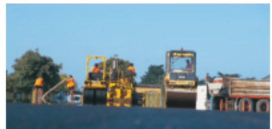
Road maintenance by Works Infrastructure
