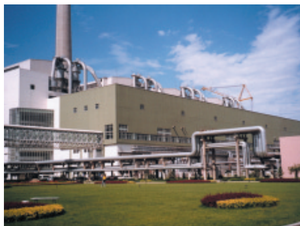
Beijing Yire Power Station
