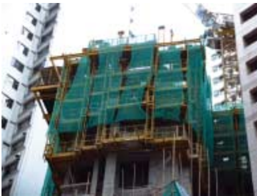
Construction of a residential project in the mid-levels
