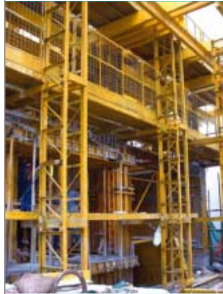
A site view of the 'slip-climbform' construction method
