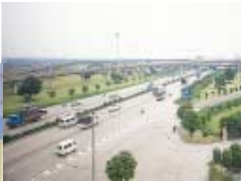
Shunde Interchange of the Shunde Roads
