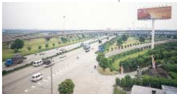
Shunde Interchange of the Shunde Roads
