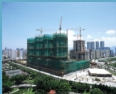
2000 to 2004 : Construction works in Progress
