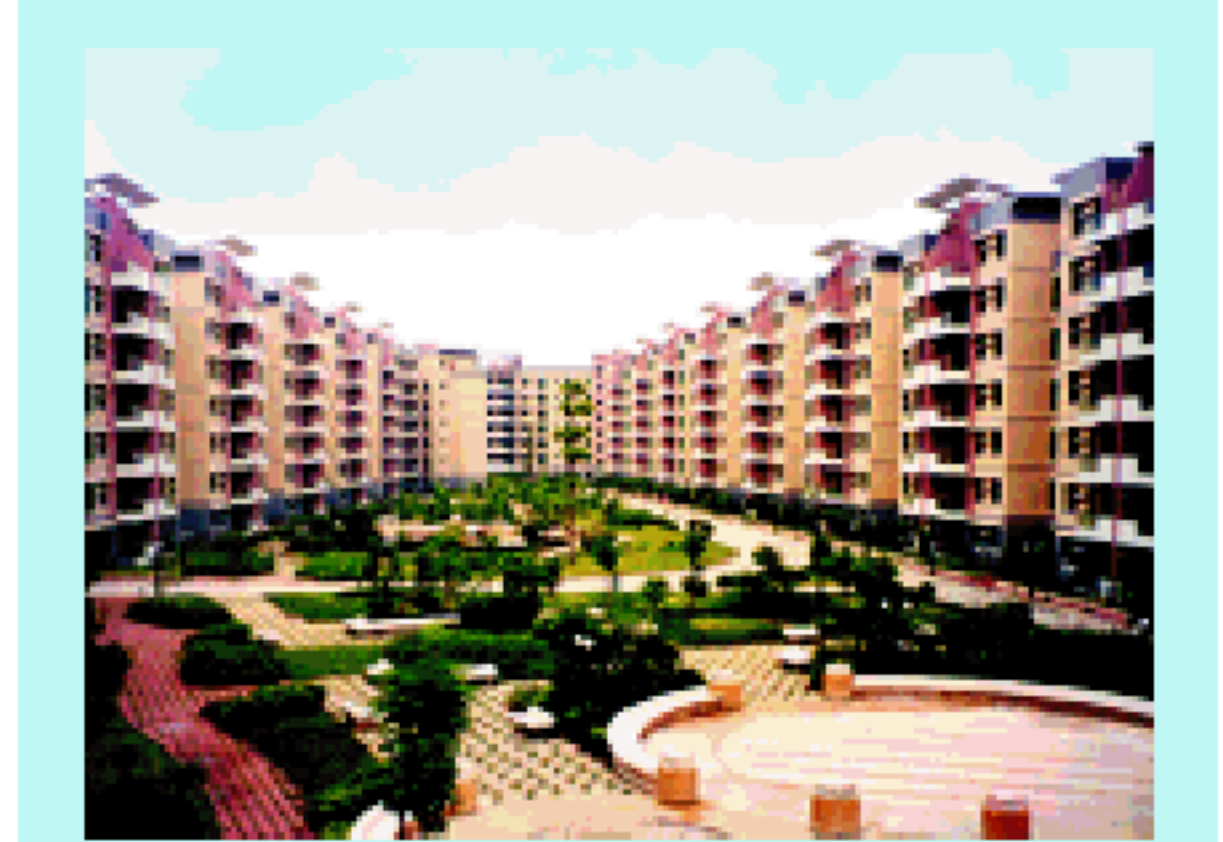
Lexi New City, Phase VII, Shajiao Island, Panyu (Fanghua Garden - Luotao Villa)
