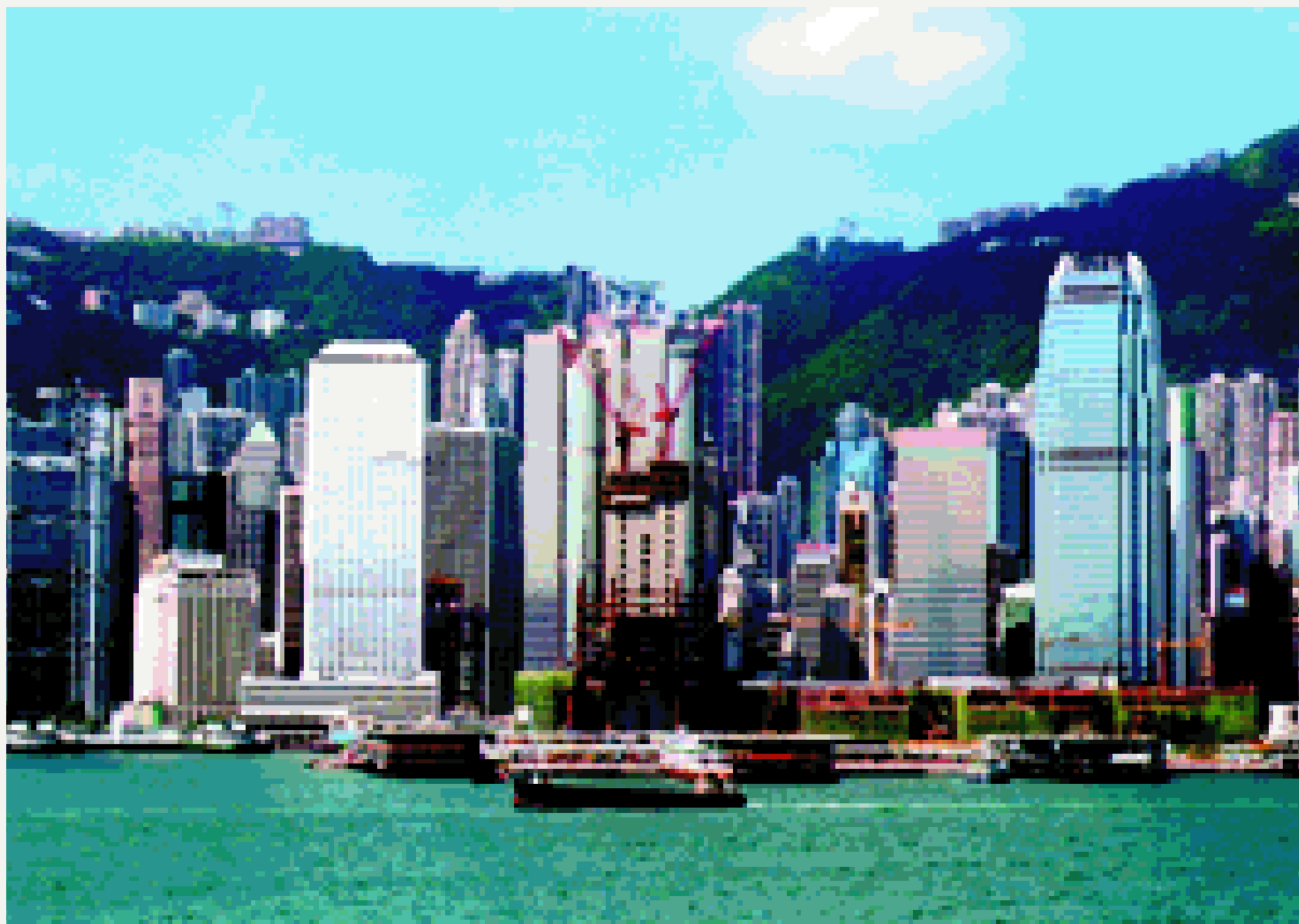
A view of the IFC project from the harbour
