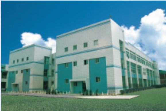
Newly constructed production facilities at Putian City, Fujian Province
