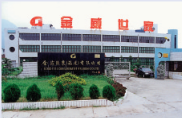
Exterior of the Group's production facilities at Putian City, Fujian Province
