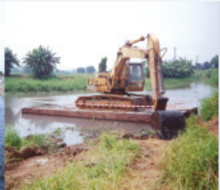
Watercourse Desilting Works in the Territory and Auxillary Works under the Drainage Ordinance
