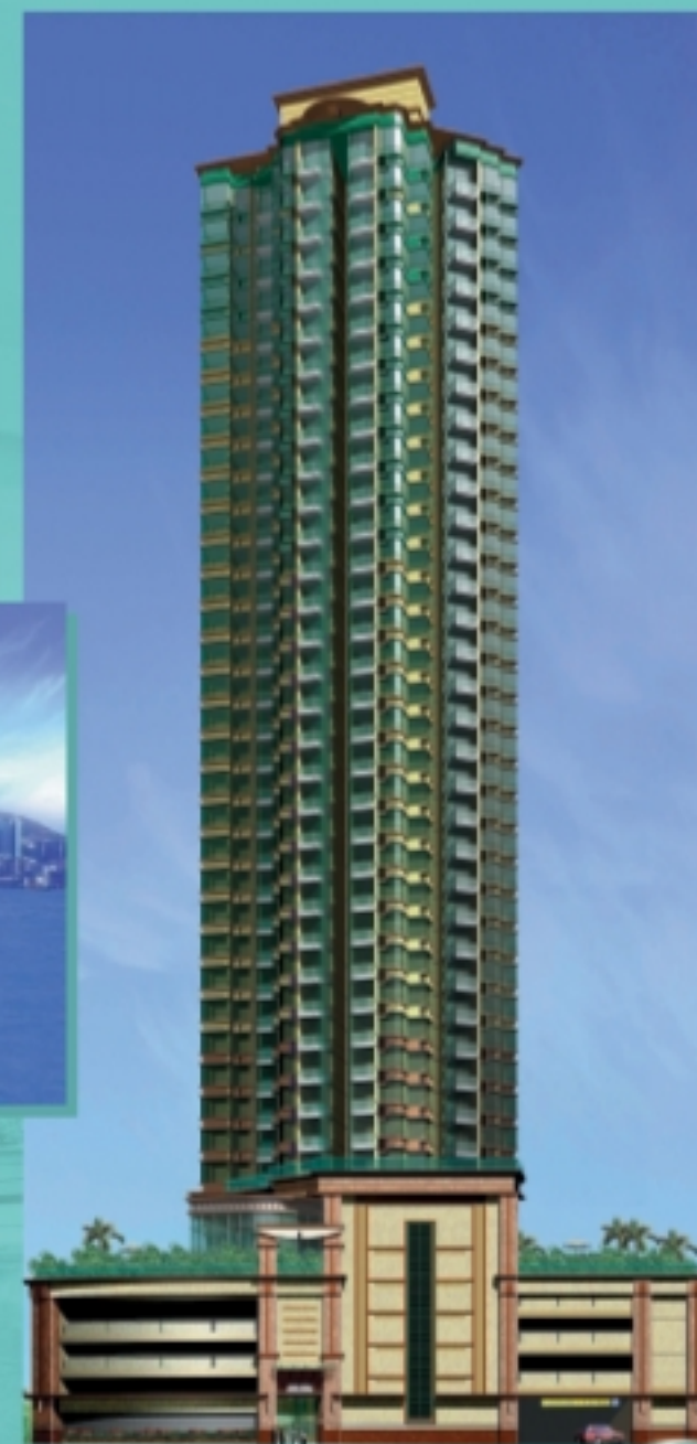
The Oakridge at Yiu Hing Road, Shaueiwan 筲箕灣耀興道星河灣
