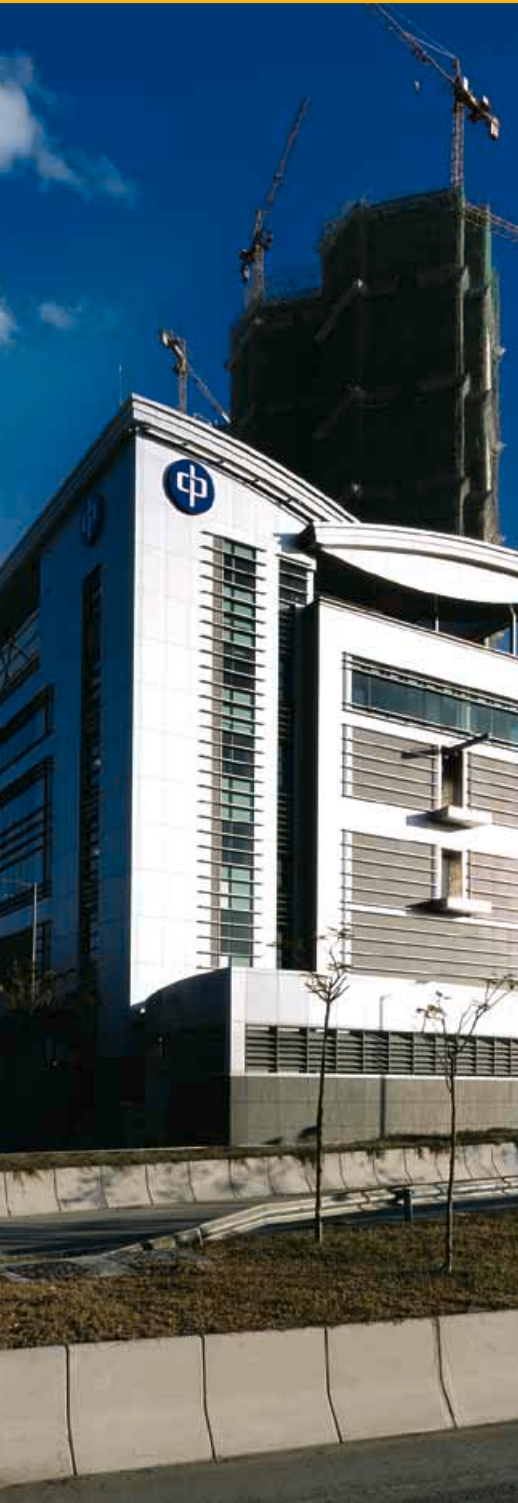
CLP Centenary Substation in West Kowloon
