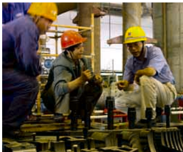
Installation work at Heze II Power Station Unit 3, Shandong
