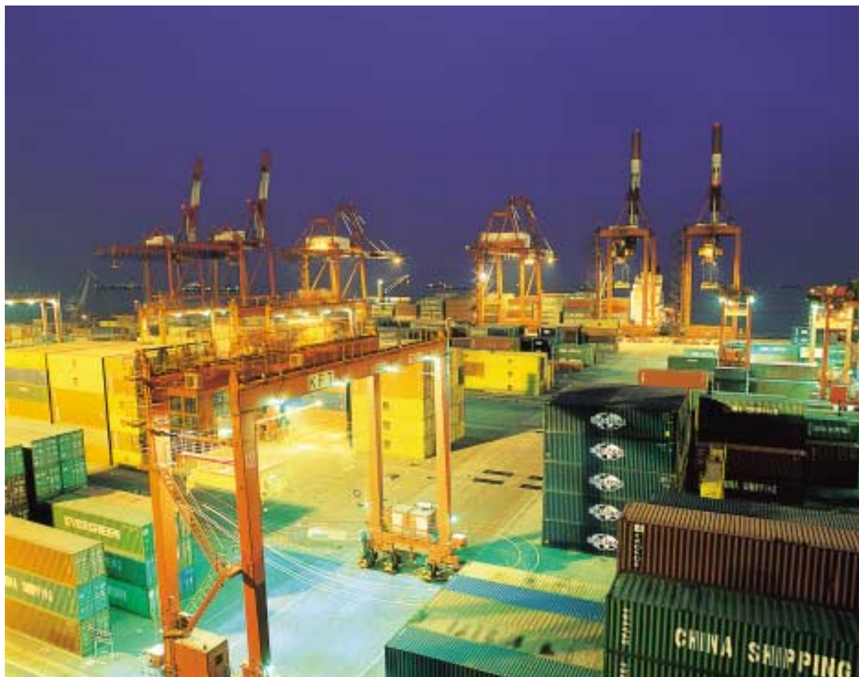
New berth at Shenzhen Kaifeng Terminal, Shekou, Shenzhen, PRC
