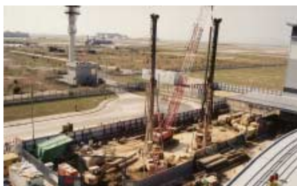
Construction of Western By Pass at Asia Airfreight Terminal
