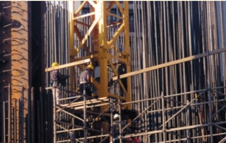
Comprehensive Redevelopment, Mongkok – Construction proceeding at full speed
