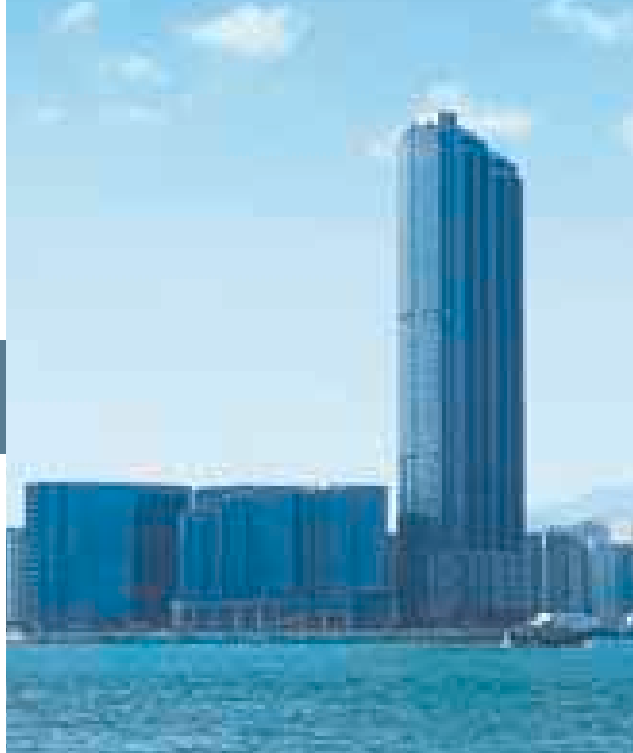
An imposing 72 storey development on the Hunghom waterfront, The Harbourfront Landmark is the highest waterfront residential building in Hong Kong.
