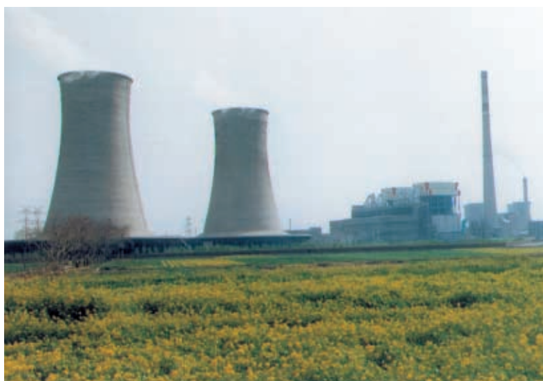
Henan Power Plant
