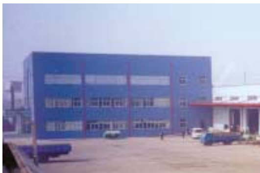
The warehouse in the Jiuting Industrial district, Shanghai has a gross floor area of 17,474 sq.m.
