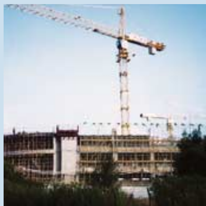
Daido Superslab used in ArchSD school project at Po Kong Village Road
