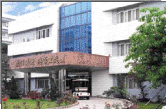
Central Administration Building
