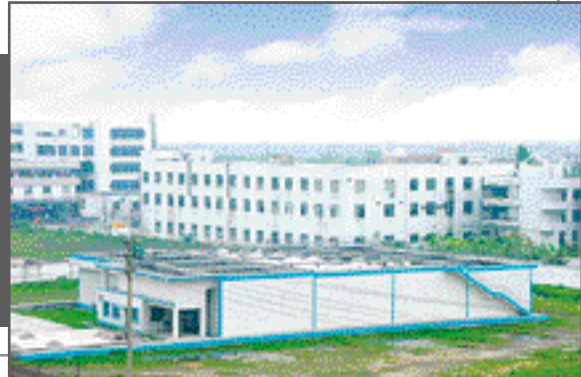
Sewage Treatment Plant
