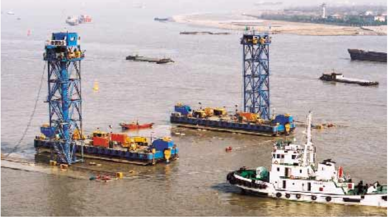
Marine Works-Towing and Sinking Preparation of Element 沉埋管的拖運及沉放準備工作
