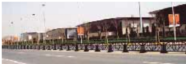
West Elevation of Exhibit Halls (Far View)
