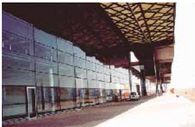
Steel Structures for Exhibit Halls
