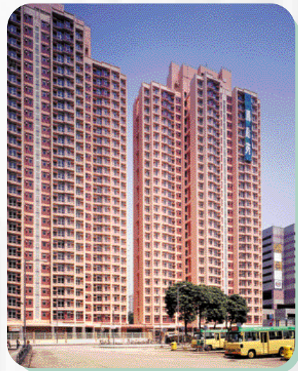
Construction of HOS Development at Fung Cheung Road, Yuen Long
