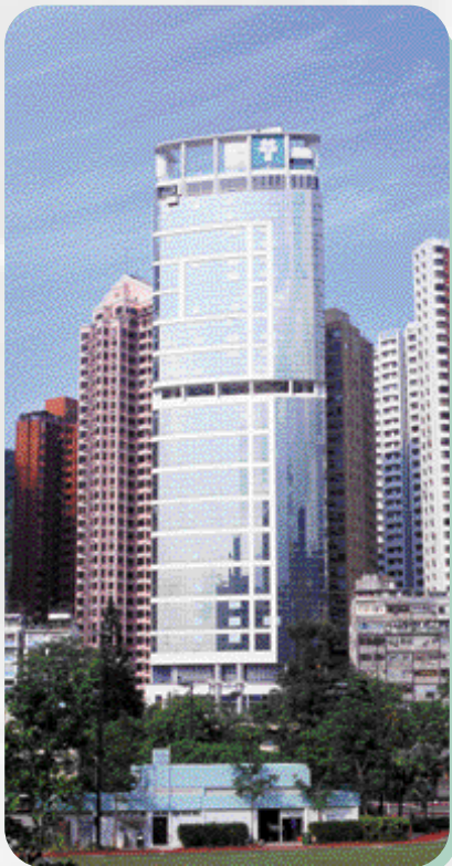
Hotel Development at 148-160, Tung Lo Wan Road
