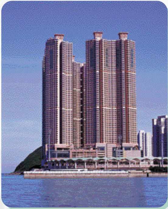
Superstructure for Commercial/Residential Development at C.W.I.L. 152, Siu Sai Wan
