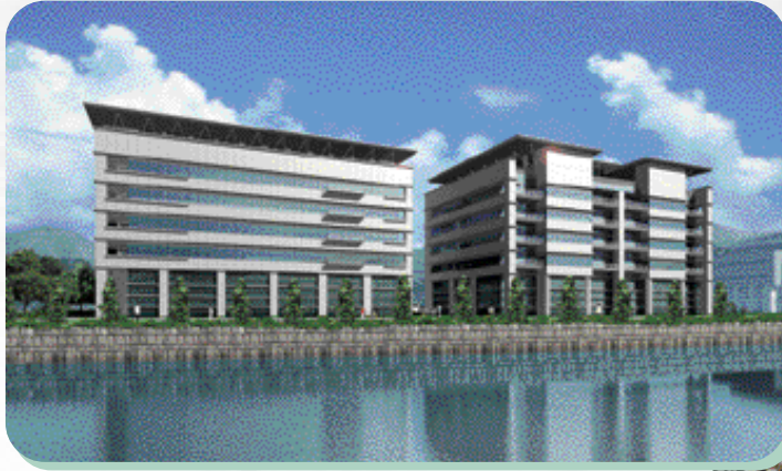
Construction of Building 4 Science Park at Pak Shek Kok, Phase 1b
