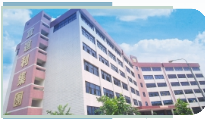
Main Factory in China
